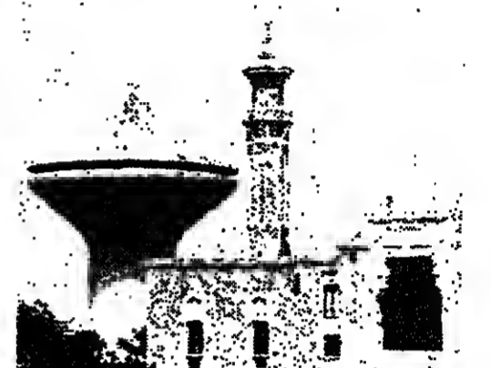
The Jeddah Water tower. See page 7 for article on agriculture and water supply
